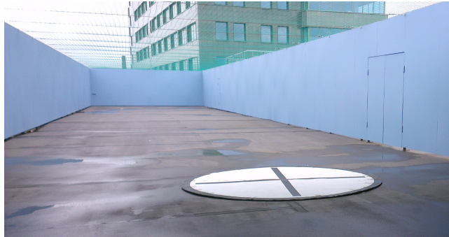
Figure 2: Corridor with landing zone circle
