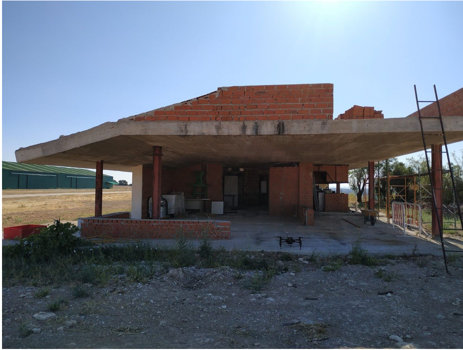
Fig 8: Entrance of the house for delivery of fragile package
