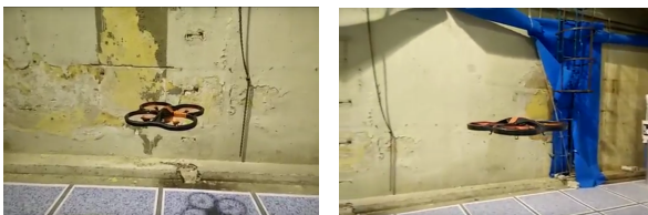
Figure 10: The aerial robot (AR Drone 2.0) during wall inspection.
