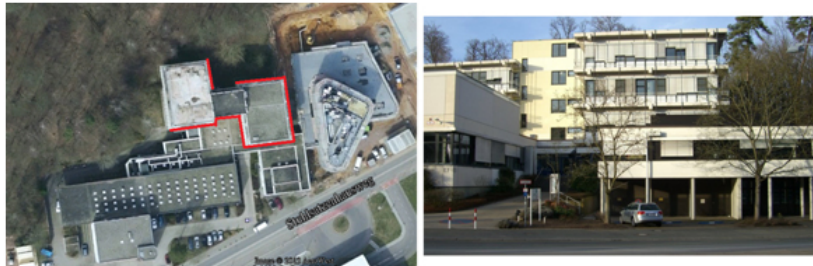
Figure 2: Left: Aerial view of Fraunhofer IZFP with rendered line indicate inspection facade. Right: Front view of the Fraunhofer IZFP.
